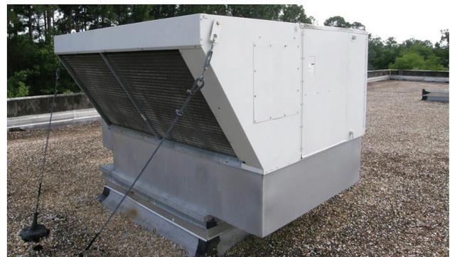
chillers produce cold water, which is pumped to one or more air handlers or fan coil units throughout the building, where the water absorbs heat from warm indoor air. The cool air is then distributed around the building through a network of ducts. Water-cooled chillers, which use a cooling tower to remove heat, are typically more efficient than aircooled chillers, which blow air across the condenser coil.
