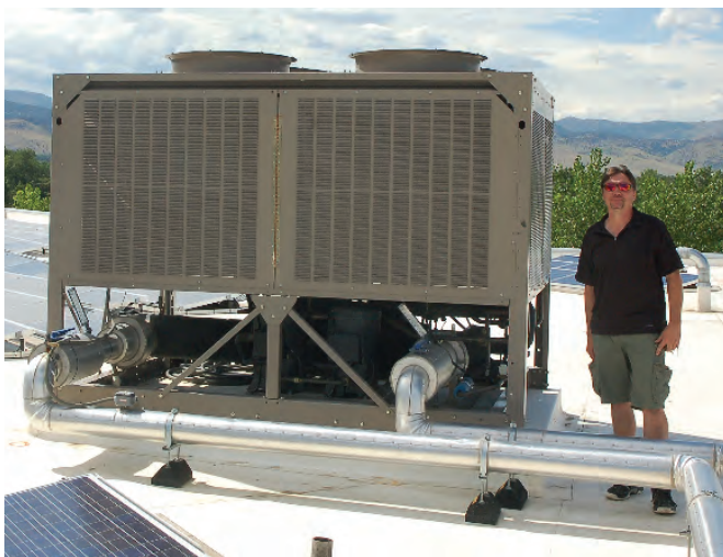
Figure 1: 40-ton air-cooled chiller. Air-cooled chillers use fans to reject heat by drawing air across the condenser.
