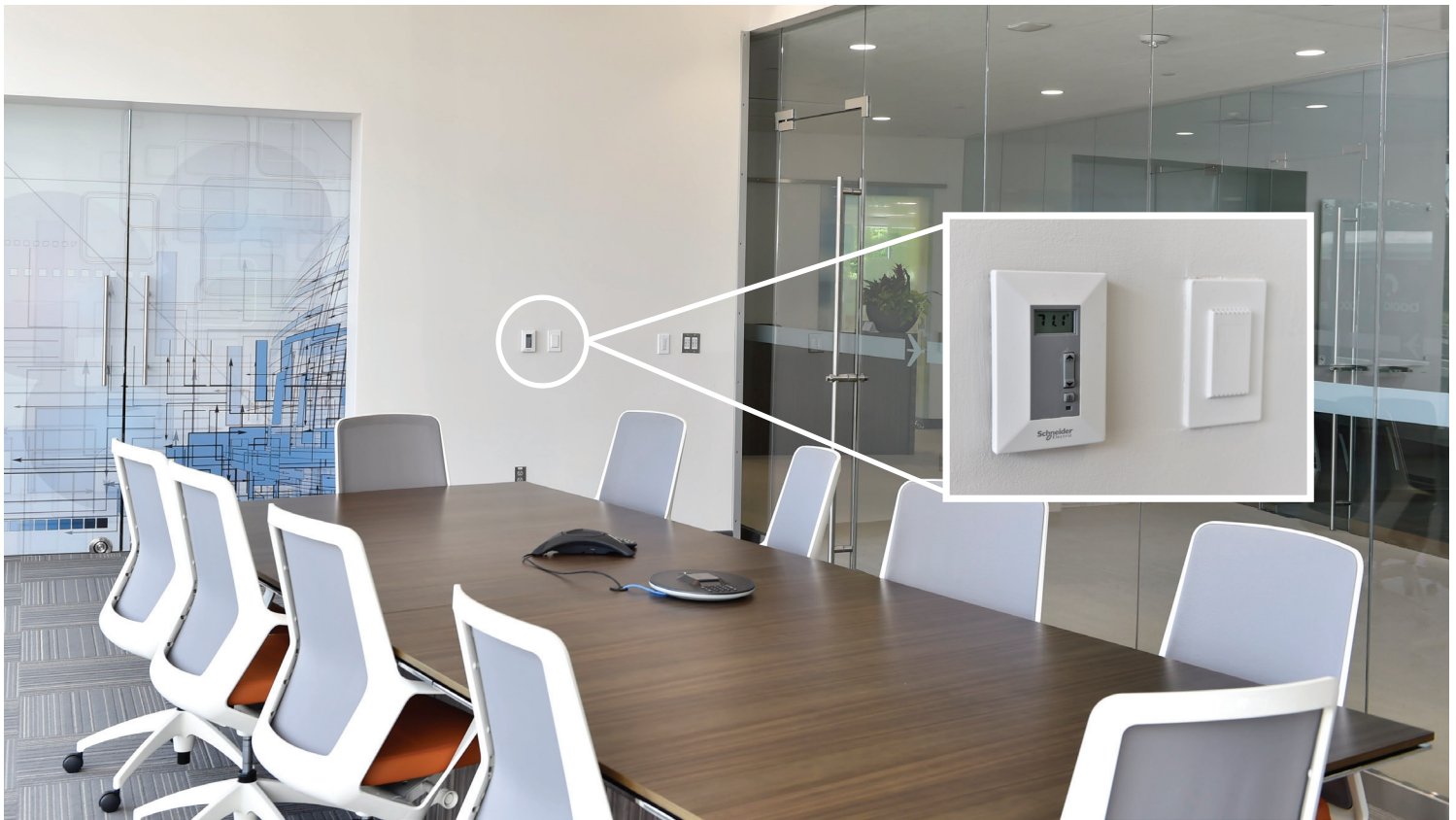
A DCV sensor (on the right) can easily be added to your existing Heating Ventilation Air-Conditioning (HVAC) system and is typically located next to a thermostat.
