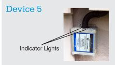
Two lights located on the top of the device.
